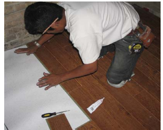
Installing ClickSealed plank by the bar
