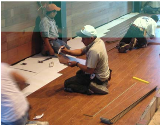
Applying ClickSeal on the stage
